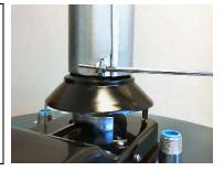
Using a #2 Philips, remove draft divert (black hood cap) from the damper housing. Set off to one side on top of the water heater.
