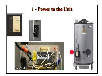
A normal 120 VAC circuit is connected to the water heater; black to black, white to white and green to ground. IF you have power to the machine, and the transformer is working, the green LED label **POWER** will be on.
