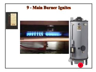
The main burner lights and begins to heat the water in the tank.
