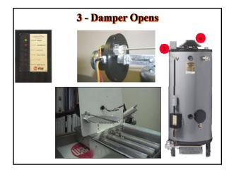
The blue wire provides power to the damper motor that drives the damper blade open. The damper blade, being open, will allow combustion gases to escape through the venting.
