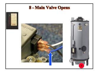
After the pilot is lit and recognized by the electronic control, the ignition control module energizes the main valve.
