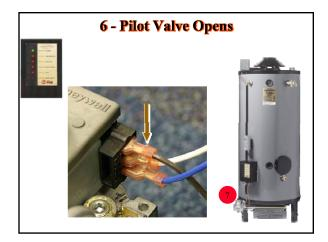
The spark ignitor will continue to spark for 90 seconds; then stop.
