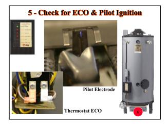
The control module attempts two events simultaneously. The ignition control module generates a 10,000 volt spark at the pilot electrode assembly and attempts to light the pilot. You will hear a distinctive 'clicking or arcing' noise.
