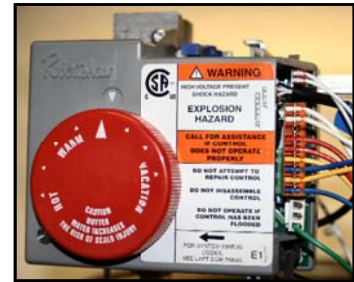
Figure 4 – FV Wiper Gas Control
