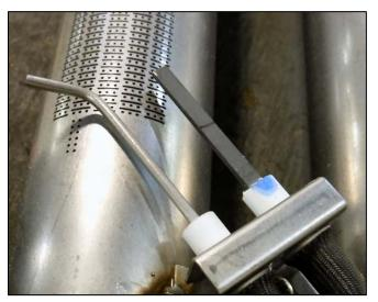
Hot surface igniter should extend over closest row of burner tube holes.
