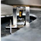
7. If the assembly has been activated, then the bulb is missing. You will also see the damper rod penetrating into the assembly.
