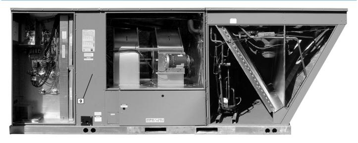
A control box component location legend sticker (10) is located on the left interior surface of the control section to match the components to the wiring diagram for ease of trouble shooting. Wiring is numbered on each end of the termination and color-coded to match the wiring diagram. The control transformer has a low voltage circuit breaker that trips if a low voltage electrical short occurs. There is a blower contactor and contactor for each compressor.
