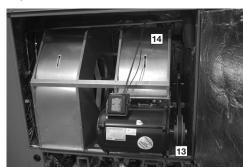
screw, which can score the shaft, creating burrs that make blower-pulley removal difficult.
