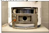
This will allow the top of the burner to clear the combustion chamber opening.
