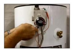
Any gasket removed from the burner assembly must be replaced with a new gasket.
