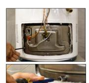
Any gasket removed from the burner assembly must be replaced with a new gasket.
