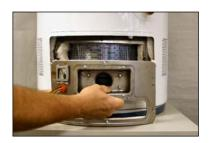
Any gasket removed from the burner assembly must be replaced with a new gasket.
