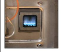
ECO is monitoring water temperature. Trips at 199°F.
