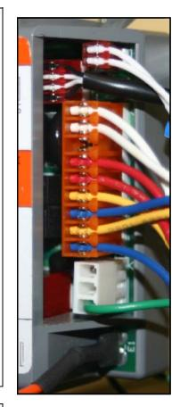
In normal operation, the switch is OPEN at beginning of call for heat. If no blower motor, then check: 120V power at the #5 yellow wire Vacuum switch tubing Vacuum switch Vent over-temperature switch is not activated If vacuum switch has failed in the closed position, the control attempts to open the switch by cycling (turning off blower, then on) the blower motor. After 5 cycles (attempts), the control will lockout. LED code is 3/1.
