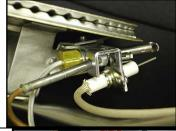
8. Install new gasket. Place burner in combustion chamber. Reinstall the four tamper resistant screws to the door assembly. Do not over tighten the screws.
