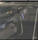
11. Check main supply tube and pilot supply tube at the gas control valve for gas leaks with a soap and water solution. Bubbles indicate a leak. Tighten all connections if a leak is found.
