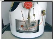
4. When the water is drained, unscrew the gas valve. It should loosen counter clockwise as you are looking at it.
