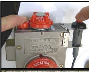
12. Set red temperature dial on thermostat to a safe position not to exceed 120 degrees.
