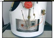
11. Tighten the main burner supply tube, pilot supply tube and thermocouple connection to the gas control valve. Connect the orange ignitor wire to the piezo striker.
