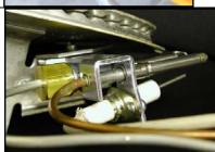
10. Clean and remove the old gasket. Install new gasket. Place burner in combustion chamber. Reinstall the four retaining screws to the door assembly. Do not over tighten the screws.
