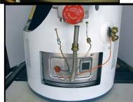
9. Tighten the main burner supply tube, pilot supply tube and thermocouple connection to the gas control valve. Thermocouple should be no more than one quarter (1/4) turn beyond hand tight.
