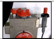
2. Remove old piezo ignitor striker by detaching the wire and prying the striker away from the gas valve.
