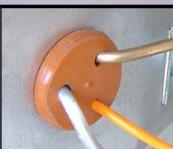
9. Reattach the pilot/electrode assembly to the burner plate.
