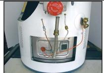
9. Reinstall the gas line to the valve. You will need pipe dope suitable for gas supply (or other sealer required by local code) on the black pipe connection to the gas valve.
