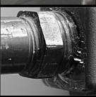
12. Look thru the sight glass to visually verify the thermocouple is enveloped in the pilot flame. Replace jacket door.
