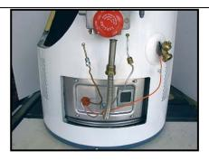
7. Turn gas supply back on. Relight pilot per the lighting instructions and turn gas valve to ON.
