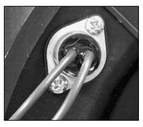
Figure 6 - Vent Over Temperature Safety Switch
