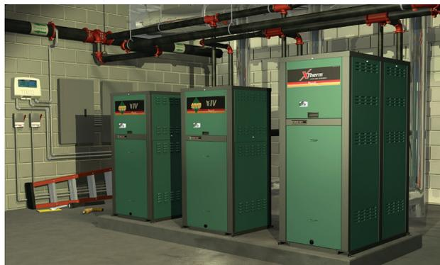
Hybrid system using 2-MVB's and 1-XTherm
