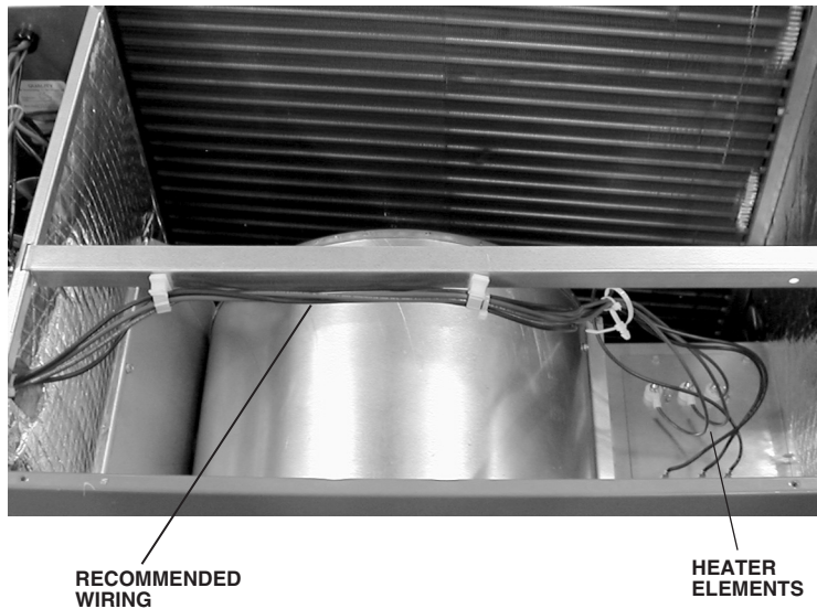
FIGURE 5 HEATER KIT INSTALLATION
