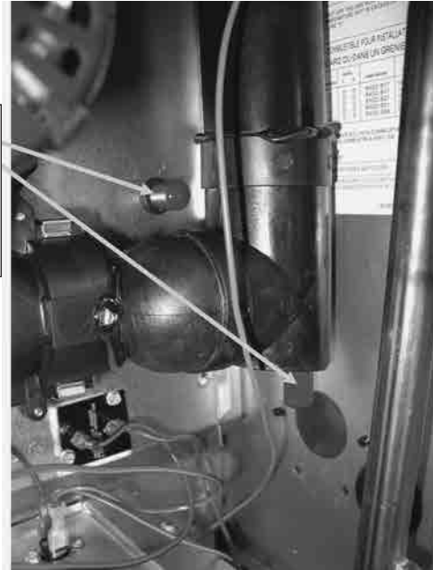
FIGURE 38 REMOVE VINYL CAPS BEFORE INSTALLING THE DRAIN SYSTEM. (-GJF MODELS ONLY)
