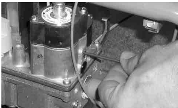
FIGURE 51 SOLENOID CONTROLLED GAS VALVE PRESSURE ADJUSTMENT ( \frac{3}{32} " ALLEN WRENCH) (FUEL CODE HH OR HG)
