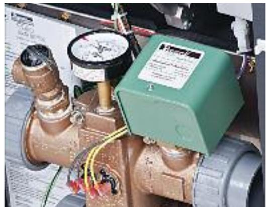
Flow switch, PRV and T&P gauge-standard
