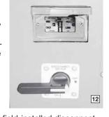
block. The suggested mounting for the field-installed disconnect is on the exterior side of the electrical control box.
