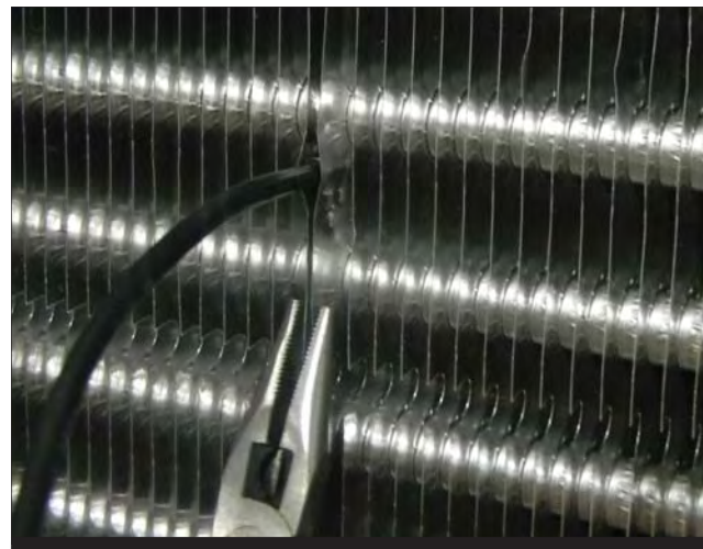
Figure 5 - Proper Sensor Positioning
