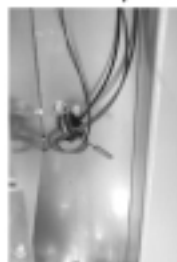
Discharge Air Sensor
