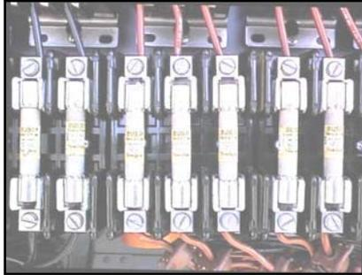
Remove the fuse from the fuse block. Set the multimeter for continuity and check the fuse. If there is continuity, then the fuse is good. If there is no continuity, then the fuse is blown and must be replaced.
