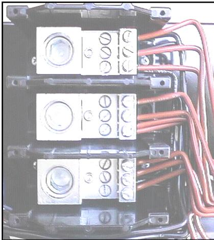
The field wiring block is the attachment point for the incoming electrical current. Line voltages may range from 208V to 480V, single phase or three phase. The figure at the left shows a three-phase configuration. You can tell it is three phase because each wire is attached at a different screw terminal on the wiring block. If all the wires were grouped together (all the red wires and all the black wires) and attached at the larger hex screw terminal, you would have a single-phase configuration.
