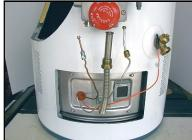
11. Turn on gas and gas valve. Relight the pilot per the lighting instructions. Turn temperature up high enough to light the main burner. Allow main burner to burn for 10 minutes to ensure air shut off plate is open.
