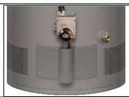
3. Remove the four tamper resistant screws at the corners of the burner. You will need a #20 size TORX head tool. Disconnect main burner supply tube, pilot supply tube and piezo ignition wire.
