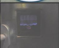
12. Reset thermostat to safe setting. Rheem recommends no hotter than 120 degrees.
