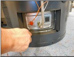
4. Remove burner access door. Remove the old door gasket. Clean metal surfaces.
