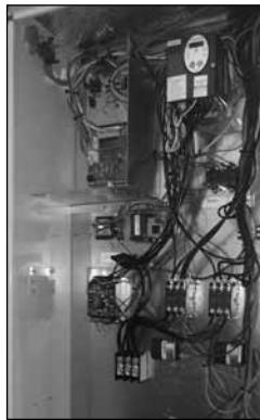
For added convenience in the field, a factory-installed convenience outlet (**13**) is available. Low and High voltage can enter either from the side or through the base. Low-voltage connections are made integrated cooling control. The high-voltage connection is terminated at the number 1 compressor contactor. The suggested mounting for the field-installed disconnect is on the exterior side of the electrical control box.
